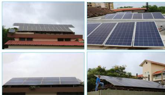
The fleet of Roof-Top SPV systems powering Street Lights on Campus: (Clock-wise from top left) Rooftop 3.6 kWp SPV System on PCC-1, Rooftop 6.0 kWp SPV System on PCC-2, Rooftop 6.75 kWp SPV System on PCC-3 and Rooftop 4.5 kWp SPV system on PCC-4
