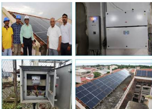
Functional Sub-systems: (Clock-wise from top Right) System Investigators, Three-Phase Inverter (100 kWp), View of Longest String Array of SPV Modules and Bi-directional Energy Meter for the Grid-tied System in 33 kV Sub-station.
