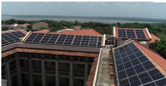
An Aerial View of the Roof-Top Solar Photovoltaic System (100 kWp) installed in the A-Wing of the Institute Building (courtesy: Drone Photography by M/S Revayu Pvt Ltd. New Delhi)
